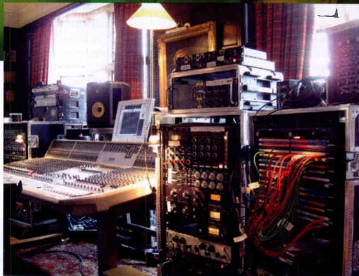
Genzo Townshend's rolling Electric Landlady Studio can be set up wherever a client wishes.
