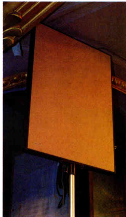
One of the NXT flat panel speakers used for the surround system
