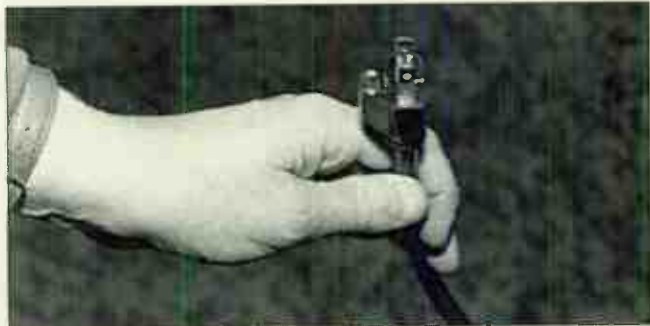
PHOTO 1: Beware of missing grounding plugs.
