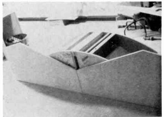
Going back in time, here's a photo of the Paragon enclosure before top sections and the refractor panel were added.
