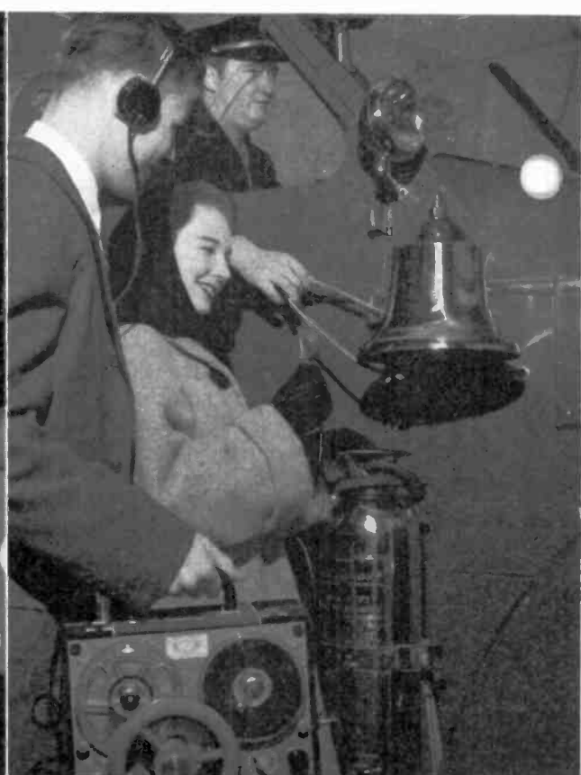
Scavenger hunting for sounds with a portable tape recorder is a new game that you can spring on your guests. It's much more fun than scavenger hunting for objects. The portable recorder shown here is a self contained unit that operates from batteries for the electronic functioning and a spring wound motor to provide the tape transport. It is the Magnemite Model 610-SD which is made by the Amplifier Corporation of America. Left: so the proprietor thinks you're crazy when you want to record the ring of the cash register—that adds to the fun. Right: collecting the ring of a fire bell at the engine house.
