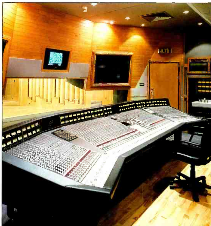
The 1000th Solid State Logic console to be built is this 72-channel SL 4000 G Plus with Ultimation in Studio One at The Town House, London. In 1978 The Town House Studios became the first studio in the capital to install a Solid State Logic B Series desk. Ian Davidson, Technical Manager of The Town House commented, 'We chose the latest G Plus console because of the commitment that SSL have made over the years enhancing and improving both the console's specification and sound quality.'
