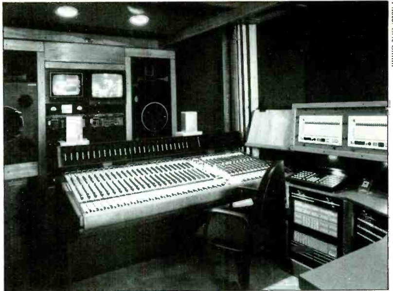
Looking towards the front of the control room over the Harrison MR4 to the customised Fostex LS-3 monitors
