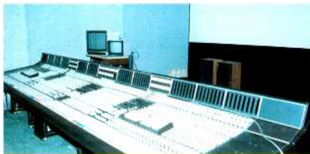
▲ Disney-MGM's SL 56124 M Series console undergoing installation and commissioning.
