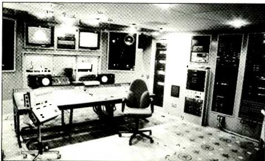
The control room
