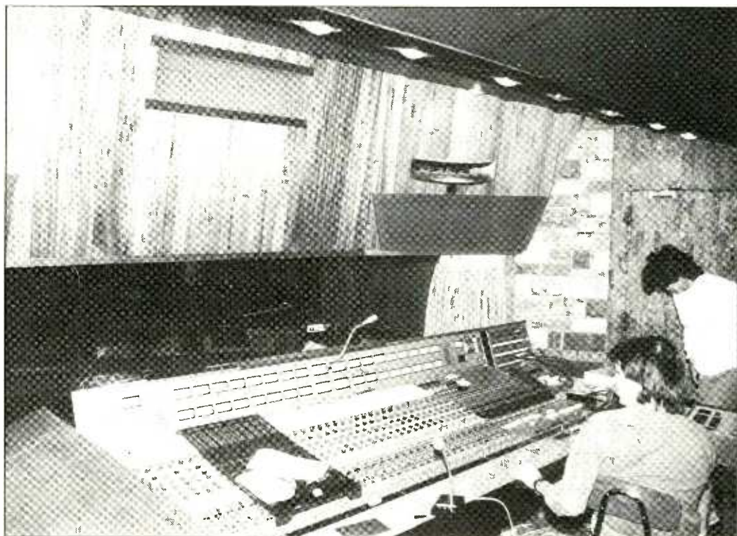
Control Room A
