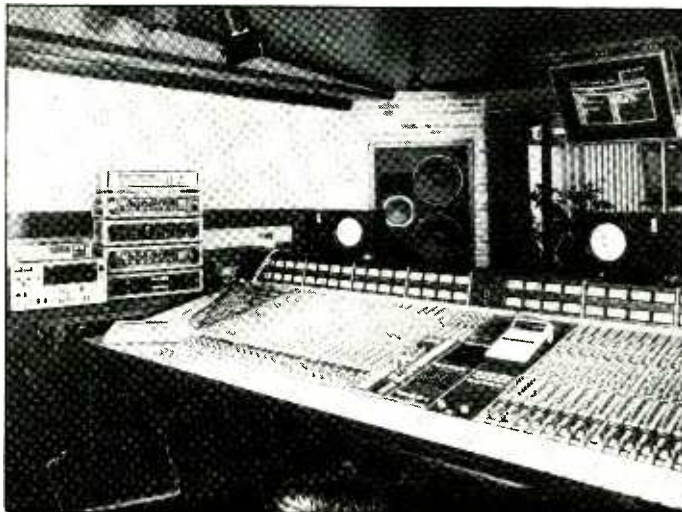
Control Room One
