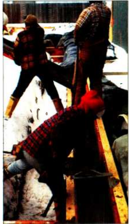
Construction continued in spite of a "typical Michigan winter."
