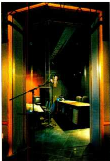
The iso booth of API provides clear sightlines from both the engineer's and production/director's chairs.
