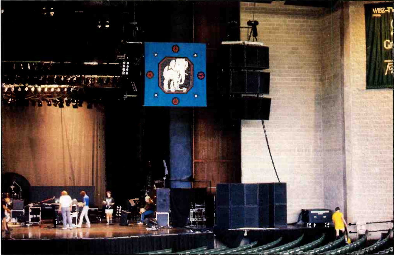
One dozen speaker enclosures were hung in left and right arrays; another dozen were stacked two high at stage level on each side.
