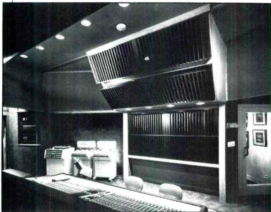
Figure 4. Custom diffusive rear wall cluster at Whitney Houston's studio. Designed by John Storyk & Associates.
