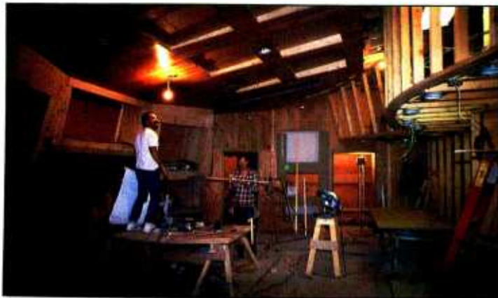
Studio A control room above, was designed and constructed with a floating inner shell on which the wood framing sits, and the concrete block sits on the structural slab. Six tons of imported hand-cut and polished Italian marble and Southern cherywood paneling were also used.
