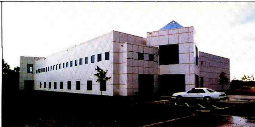
Paisley Park Studios is located on a 9½ acre site in Chanhassen, MN, a suburb of Minneapolis. The structure is a steel frame building with an aluminum covering, featuring a thermal enclosure with insulated aluminum panels, double 1-inch thick insulated glass and a poured concrete roof over metal decking for sound control.
