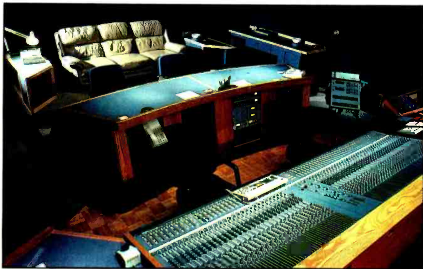
Master's Digital Mix Theatre incorporating a Soundmaster Editing System, a custom 64 input automated Neotek Elite console, variable 6 channel monitoring and twin 3324 multitracks.
