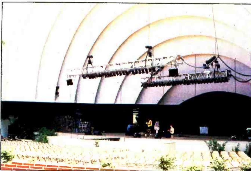
Figure 4. Front view of Waikiki Shell. Note the Meyer UPA speakers suspended from the lighting truss.
