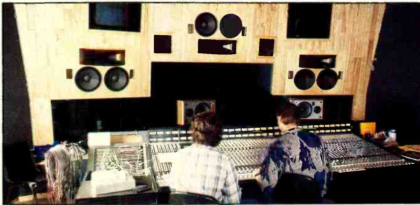
Three custom-designed Hidley-Kinoshita monitors are provided in each control room for 3-channel (left/center/right) monitoring of film and video mixes.
