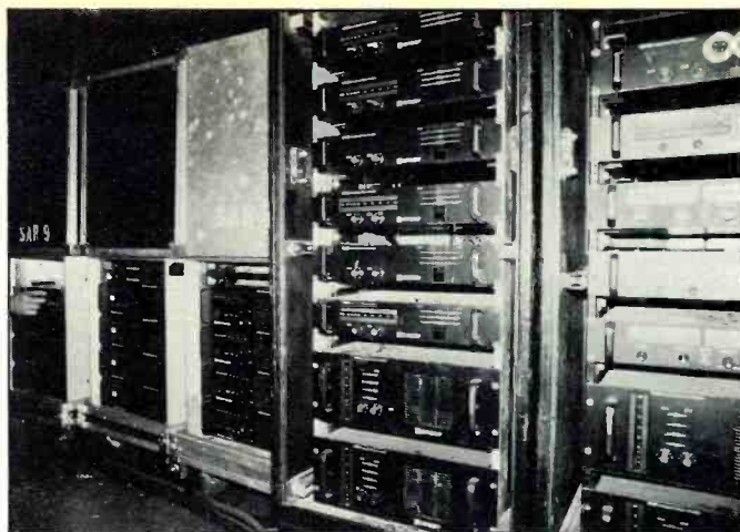
Figure 2: (Shown left) Jim Gamble Associates' HC-40-24 mixing console as supplied to the Grateful Dead by Ultra Sound. Figure 3: (Shown right) Ultra Sound packages its Crest amplifiers in two different types of racks. Four Model 4000 units are housed in compact racks, while larger systems use five Model 3500 and two Model 5000 amplifiers per rack.
