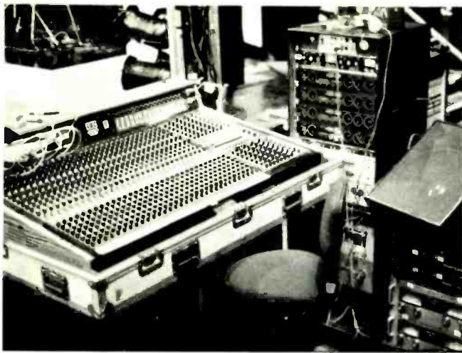
Figure 10 (shown left): The streamlined stage monitor system is centered around a Gamble SC 32-16 touring board. Yamaha F-1030 and Sundholm 202 electronic crossovers are used to offer bi-amped mixes. Figure 11 (shown right): Custom floor slants for Huey Lewis and guitarist Chris Hayes hold two JBL E-120 speakers and an Emilar driver. Sturdy bracing and a metal grill allow the performers to walk the front of the box and stand on it.
