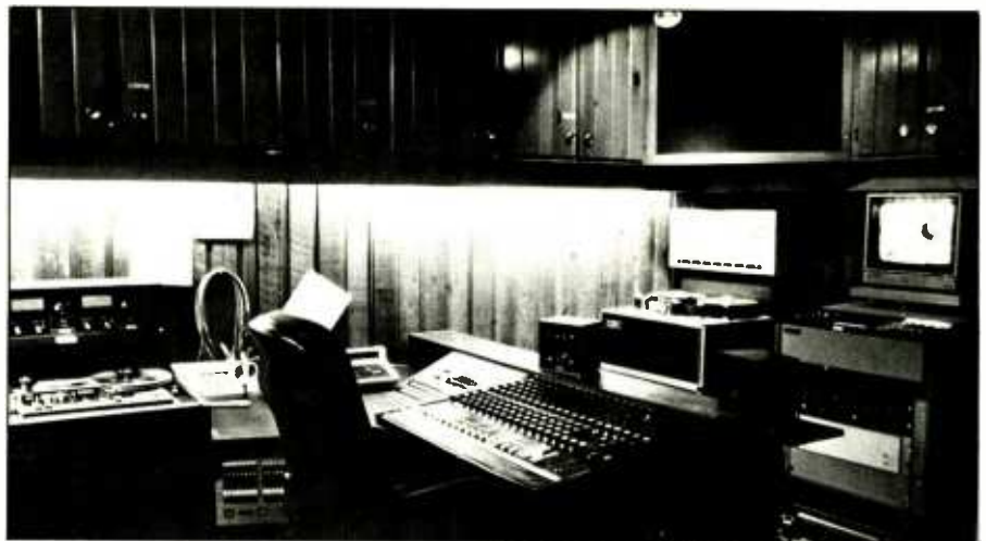
Edit One, a sound-effects suite, features an Audio Arts 16-input console, a Lyrec TR532 16/24 track, and three Scully 280B two-tracks.
