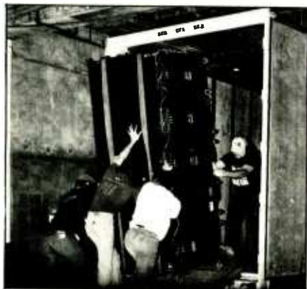
Figure 2: Enclosures are trucked in stacks of five, and secured with straps to sturdy metal dollies.
