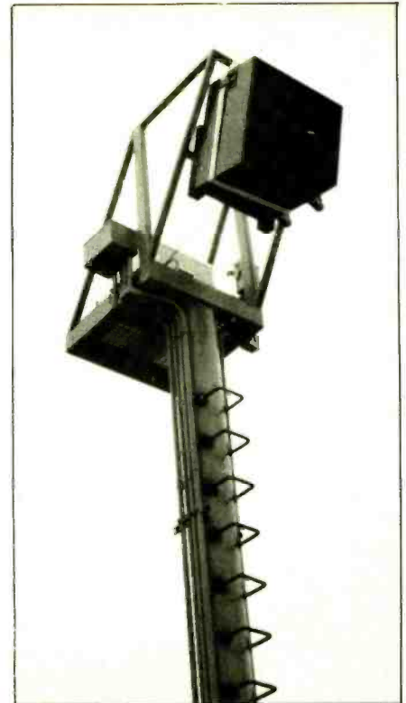
Figure 6: One of seven delay-line speaker towers serving the lawn seating area. Cabinet houses a 15-inch Fostex bass driver, and a two-inch Emilar compression driver and horn.
