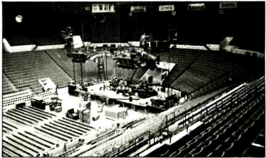
"A contemporary hanging component system used by Neil Diamond with 'constant-directivity' type horns (Stanal Sound)."
