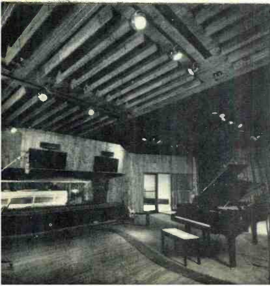
louvered ceiling, open over live area
