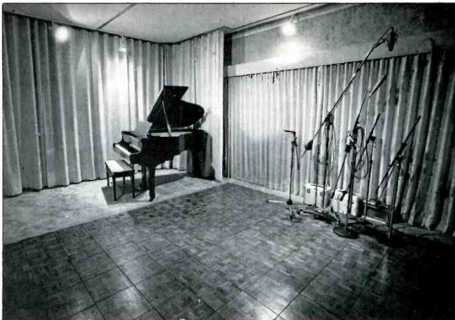
The large tracking room includes triangular redwood louvers that cover all four walls to provide non-parallel surfaces. Absorbent drapes can also be pulled across the walls to further deaden the area's acoustics.
