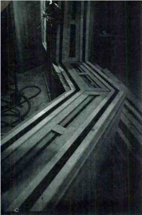
Control room window frame detail — Village Recorders, Studio D. Photo: Steve Finestone.
