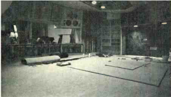
Anti-static underlay and acoustic sheathing prior to final finish.
