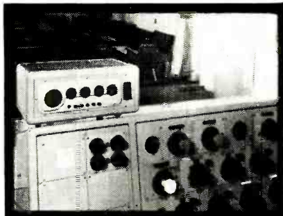
A studio control room where the programmes are passed through a QUAD control unit for special balancing.
