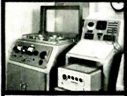
Quality Check Room. Programmes originating from abroad are here passed through a QUAD control unit and power amplifier where they are filtered and balanced for optimum quality prior to transmission.
