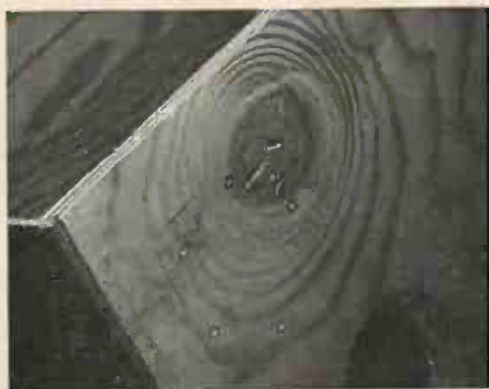
Blisters? Predrill those screw holes!
