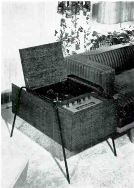
The Prades, a fine modern piece by Balladier. A combination FM-AM tuner, control unit and 12-watt amplifier is used, and a Webster player with a GE cartridge. Speaker is a separate unit.
