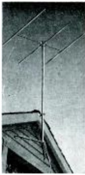
WORKSHOP FM ANTENNA AND MAST
