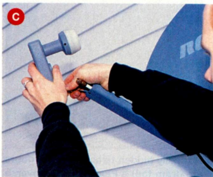
C. Nugent upgrades the DSS dish so that two different satellite-delivered programs can be watched at the same time. D. He secures the new dual LNB to the dish arm. E. He ties the phone lines from both of the DSS receivers into the main phone line.
