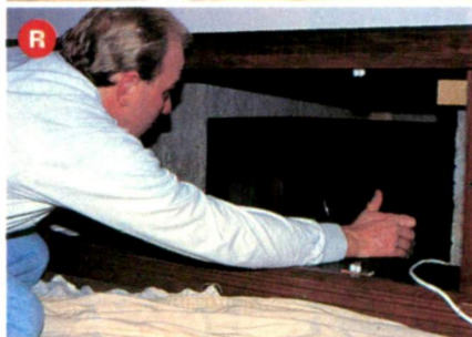
P. Placing the subwoofer on the concrete floor behind the screen prevents it from rattling the cabinet. Cables for the sub and the center speaker are tied into a neat bundle. Q. Craftsman Tom Hanff prepares an opening for the subwoofer and the center speaker in the front of the custom-built cherry cabinet. R. Julius slides the subwoofer into the cavity. S. The center-channel speaker sits in front of the subwoofer, both concealed by a black cloth grille.
