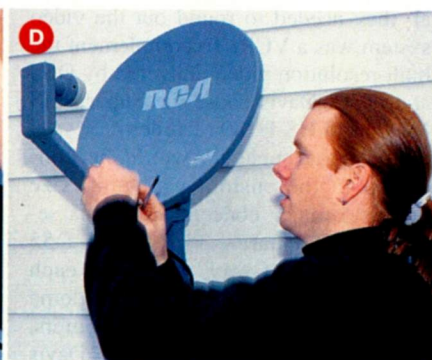
C. Nugent upgrades the DSS dish so that two different satellite-delivered programs can be watched at the same time. D. He secures the new dual LNB to the dish arm. E. He ties the phone lines from both of the DSS receivers into the main phone line.
