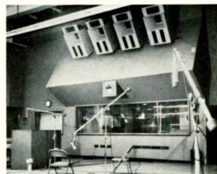
Studio A of Universal Recording Corp., Chicago, uses four Altec A-7's in monitoring 4-channel PLAYBACK .
