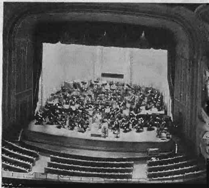
Rehearsal on the original stage set. A model of luxurious architecture, the hall produced "dry" sound because of its many absorbent surfaces.
