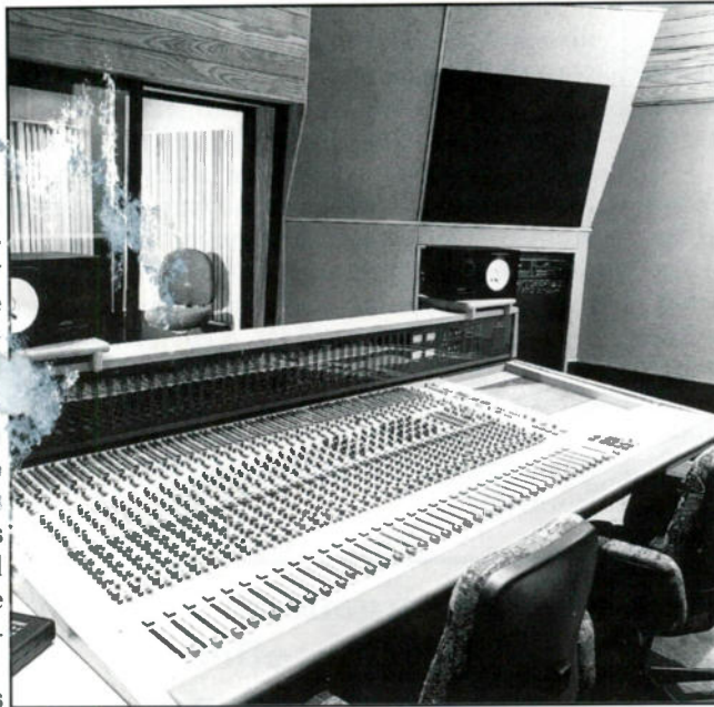
Figure 3. The Audio Post Room at KRCA-TV for mix-to-picture, post-production and is equipped with a 36-input Sony MXP-3000 console.
