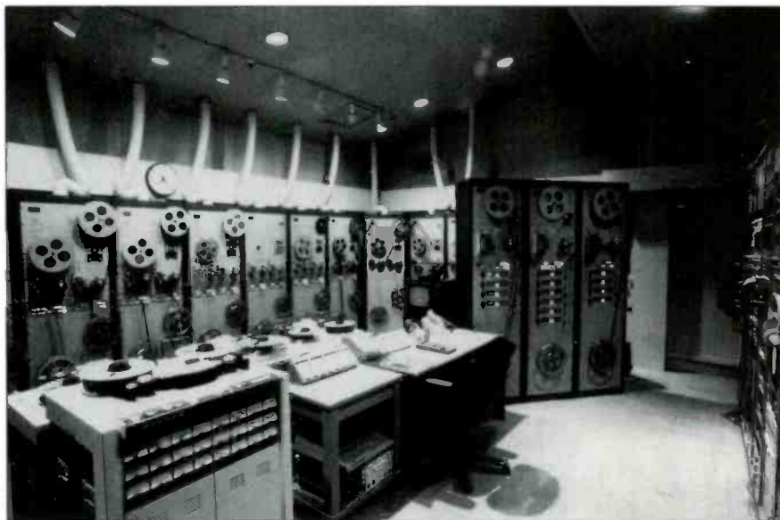
Figure 7. The Stage D machine room.
