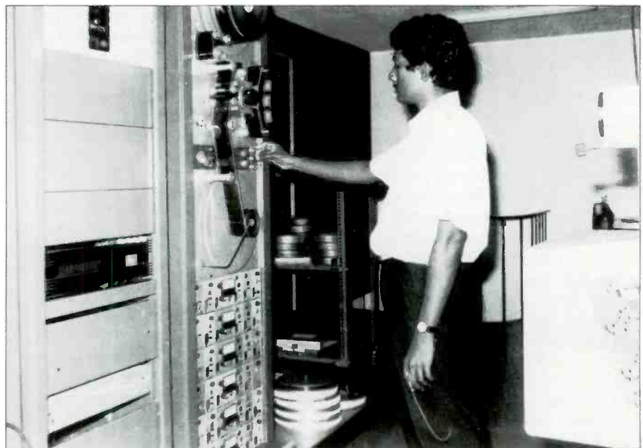
Figure 6. The transfer room is located above the machine room (next to the projection room shown in Figure 7). A trainee engineer is operating the Westrex 70 mm release print recorder.
