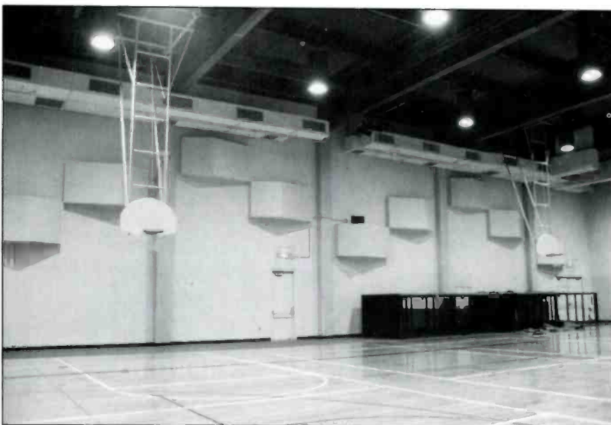
Figure 2. Wide-band diaphragmic absorbers in the gym.
