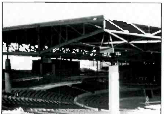
Shed at Ravinia.
