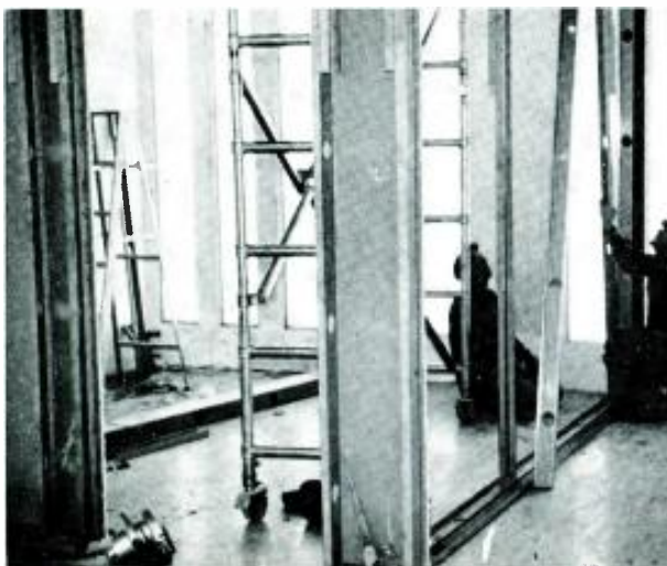
Figure 6. The double floor track into which the studs are placed.
