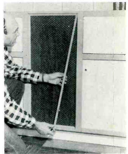
Molding is added to speaker panel.
