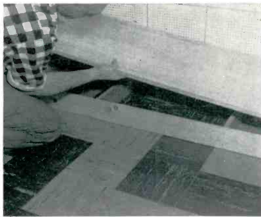
First operations in making the built-in cabinet are laying the platform, and nailing 1-by-4-inch boards to wall for top supports.
