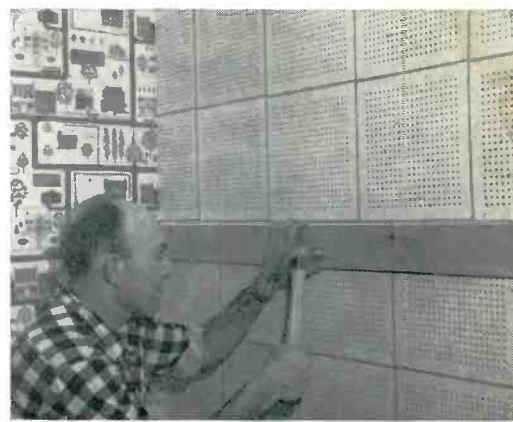
First operations in making the built-in cabinet are laying the platform, and nailing 1-by-4-inch boards to wall for top supports.
