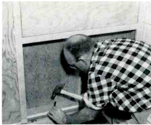
Plastic tracks for the sliding doors are nailed in place, and the record changer or turntable slides are installed on upper shelf.
