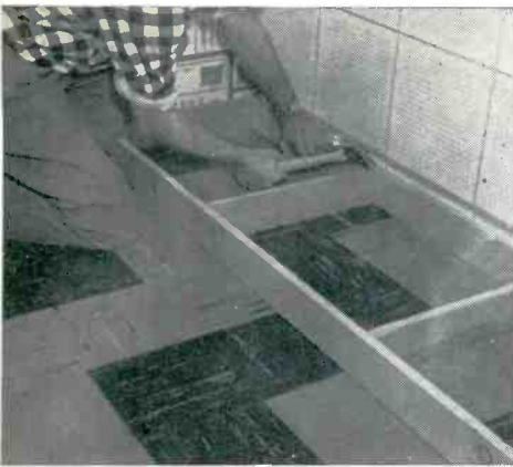
First operations in making the built-in cabinet are laying the platform, and nailing 1-by-4-inch boards to wall for top supports.
