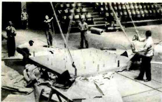
Fig. 2 —The base plane of a radial transducer is lifted into position. 15-ft. square by 9-in. thick, framed and cross-braced by 8-in. x 2-in. beams, and clad with \frac{3}{4} -in. plywood. Internally, it is filled with vermiculite and under-coated. Projections you see are \frac{1}{2} -in. steel-threaded studs and stand-off spacer bushings to support the horn flare.
