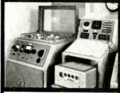
Quality Check Room. Programmes originating from abroad are here passed through a QUAD control unit and power amplifier where they are filtered and balanced for optimum quality prior to transmission.
