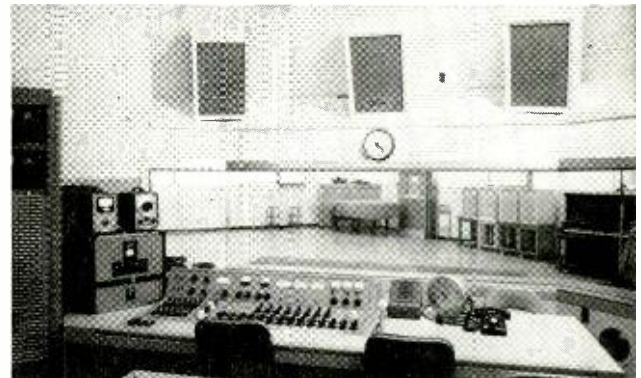
Monitoring with Altec "Duplex" speakers in Capitol's Control Room. More than 70 Altec "Duplex" speakers are used for various PLAYBACK purposes throughout Capitol Records' recording facilities.
