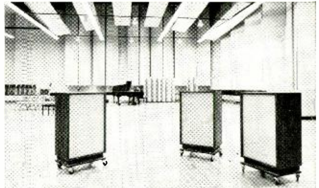
Interior of Columbia Records' Studio A in Hollywood showing CBS-built cabinets housing Altec 605A "Duplex" Loudspeakers for professional PLAYBACK .
