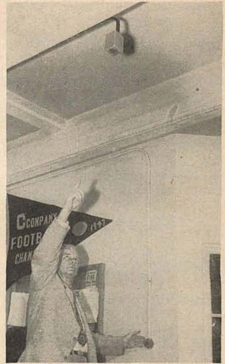
Fig. 3. Typical microphone and signal button mounting located in one of the day rooms.
