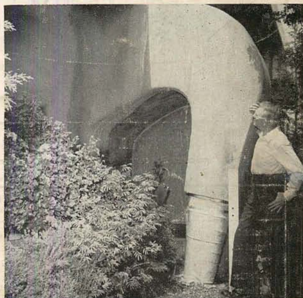
In the crusade for better bass, the music lover is likely to end up with a large exponential horn. If there isn't room for it in the house, why not build it outside? See page 17.
