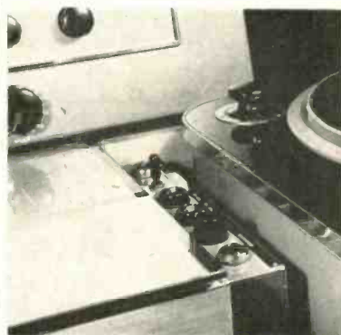
Fig. 6. Remote control box in place in one of the control rooms.
