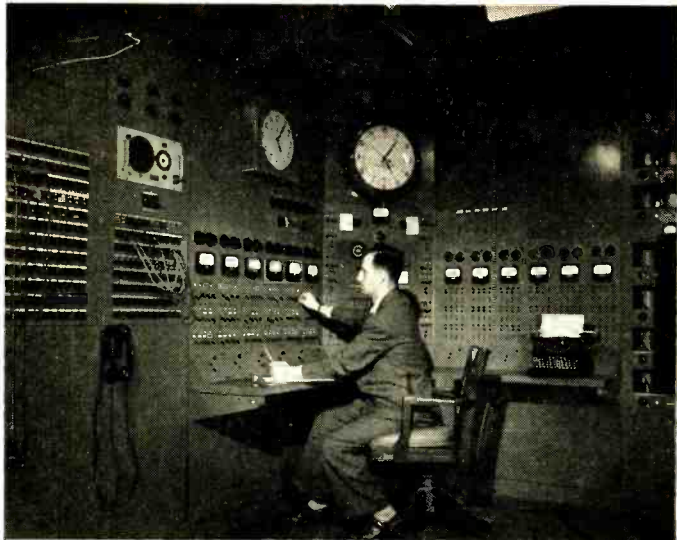
Fig. 1. An installation of twelve standard volume indicators, on an equal number of outgoing program circuits in the CBS shortwave master control room.
