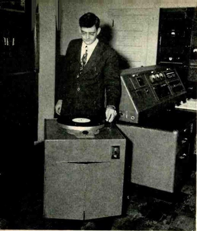
Author with the station turntable. At the left is the phasing unit of the 5-kw AM WIS transmitter. In the right foreground is the transmitter console, with a portion of the speech bays behind it.
