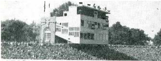
University of Michigan stadium, Ann Arbor, Mich. Altec Lansing large multicell horns driven by Altec Lansing 1/4 KW amplifier, are centralized over press stand, override noise level of 86,000 spectators. Reiss Public Address Systems, Detroit, contractors.
