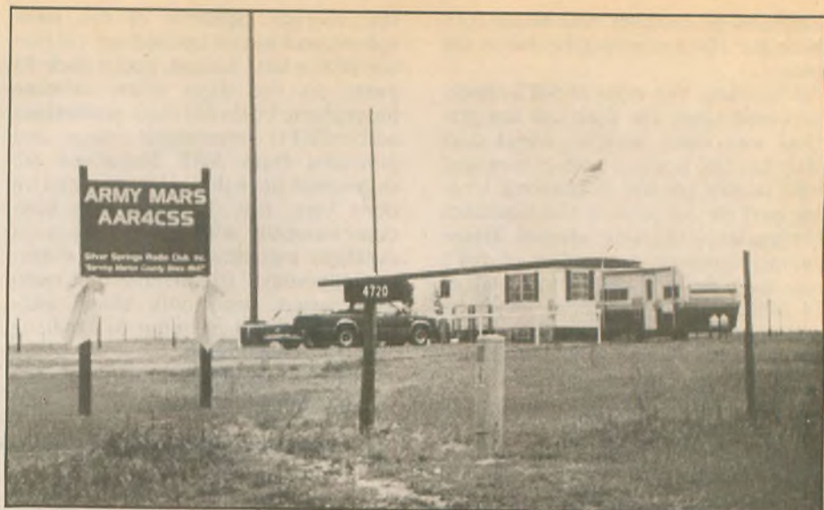
The AAR4CSS Army MARS station was completed and operational in 60 days.
