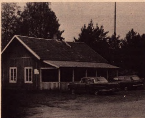
Station at Morokulien
