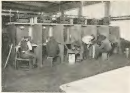
Student welders in training at General Electric Company plant
